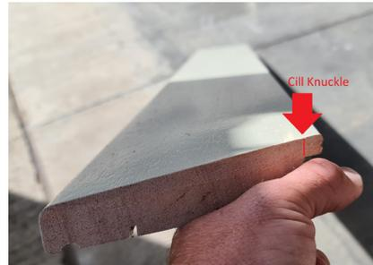
*TIP: When measuring and marking the length of the bay cill ensure you mark and measure on the knuckle of the cill extension and not the back side of the cill tongue.*
