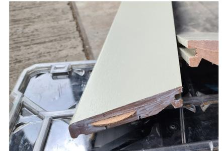
**4** Working on one piece at a time, install the cill extension onto the window (See Installing Cill Extensions section of this guide for more information). Insert the biscuit to hold the joints flush, then install the next piece of cill extension. Metal fixing plates should be fixed across the join on the underside of the cill to prevent the joint from opening up during seasonal movement.
