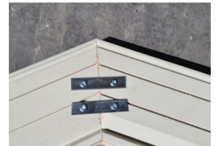
**5** The cill joint should now be sealed with opti-joint xp flexible sealant, allowed to cure for 15 minutes, and then touched up with paint to finish (paint is supplied with the original order, more can be ordered on request).
