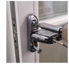
Refit the locking mechanism and any rubber infill gasket into the locking groove on the replacement sash, ensuring it is fitted the same way up as on the previous sash. Screw the handle into place and fit the screw cover caps. Screw the hinges onto the new sash, ensuring the hinge is placed in the same position as measured on the old sash to ensure correct operation of the new sash once installed. Any other additional furniture should now be refitted to the new sash.
