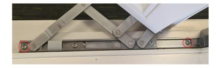
Once any screws are removed the sash is no longer fully connected to the window and must always be supported.
