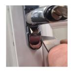
The screws holding the locking mechanism in place can now be removed, taking care to note which way up it is located on the sash. Any rubber Infill Gasket can also be removed and saved to fit into the new sash.
