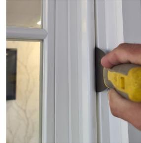
Continue tapping the knife and prising the rest of the bead to pull the fixing nails loose from the timber and release it.
