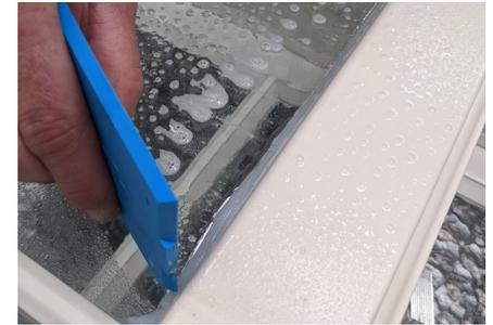
The presence of the water/ soap mix will prevent the silicone from adhering to the scraper, glass or timber and allow excess to be scraped away. Done carefully, this will leave a perfect silicone bead and create a watertight seal.
